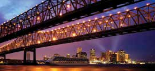
New Orleans Crescent City Bridge
