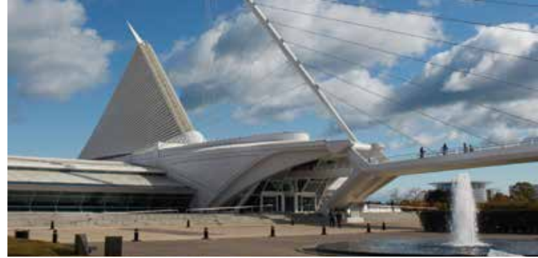
Milwaukee Art Museum (Photo Credit: Calatrava)
