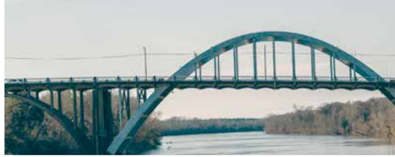
Selma Bridge Over Alabama River
