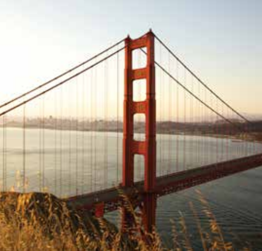
Golden Gate Bridge
