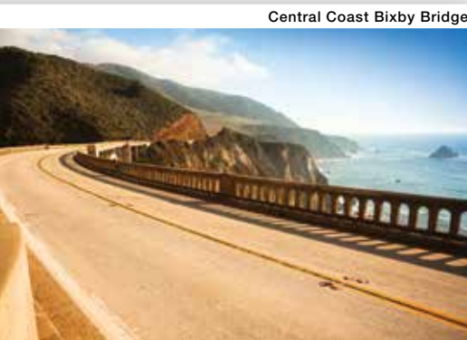
Central Coast Bixby Bridge
