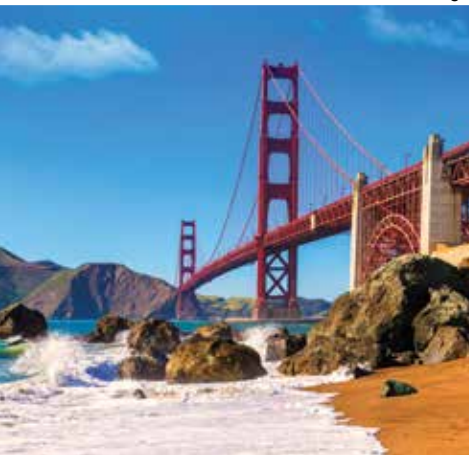
San Francisco Golden Gate Bridge
