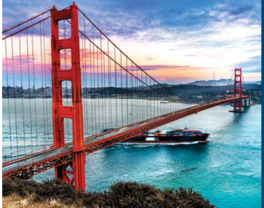
San Francisco Golden Gate Bridge
