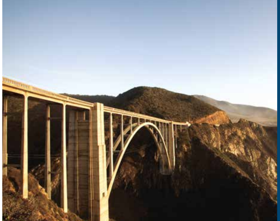
Central Coast Bixby Bridge
