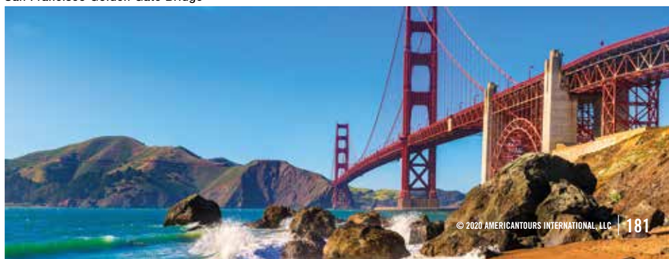
San Francisco Golden Gate Bridge
