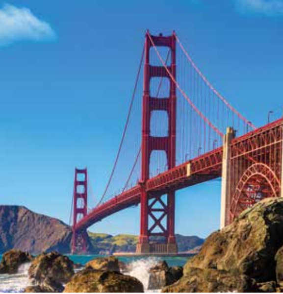
San Francisco Golden Gate Bridge
