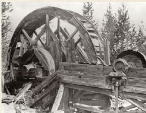
Waterwheel at Skelton Mine ca. 1930
